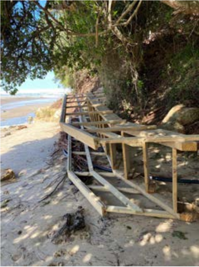
RIPPED OFF: The newly built steps the NCOA had built from the public loos to the beach broke loose in the 2023 storm surge.
