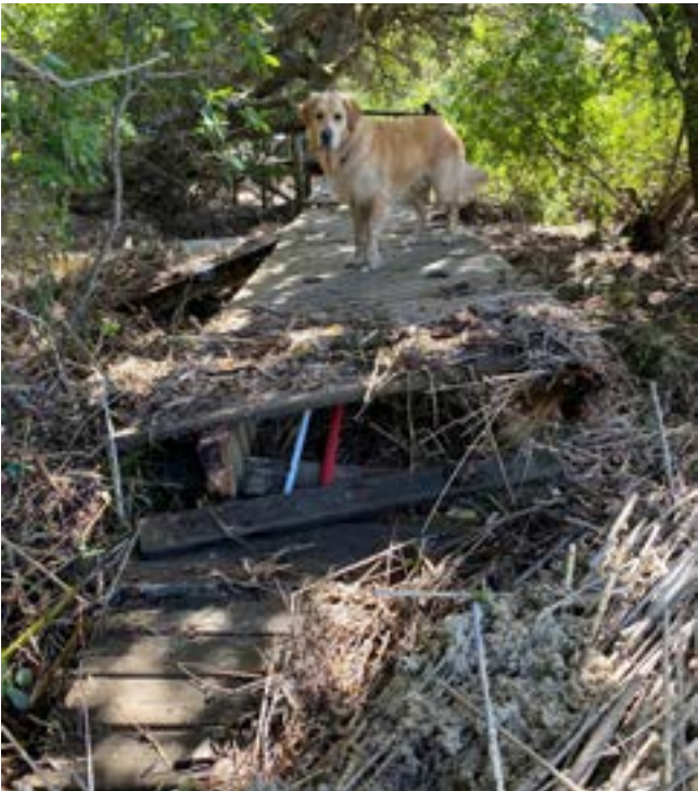
WHERE TO NOW?: The force of the 2023 storm surge waves was dissipated somewhat by the wide river estuary, but still had enough force to lift the boardwalk and move it about a metre inland.
