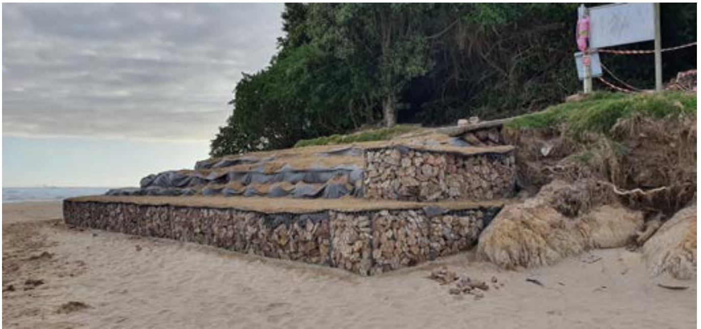
STRONGER: The vehicle ramp, which was originally just sand and sandbags, was rebuilt with two tiers of gabions to protect it against high seas and the flooding river. Beach vegetation was later planted on top to help it blend in. The new ramp stood up well to the 2024 storm surge. The NCOA applied for and was granted emergency environmental authorisation by the Department of Forestry, Fisheries and the Environment (DFFE). This rebuild was paid for by beach residents Neil and Carl Metelerkamp, Sandi Braun, the Gosling family and Derek Cockcroft - who also paid for Buccara's portion.
