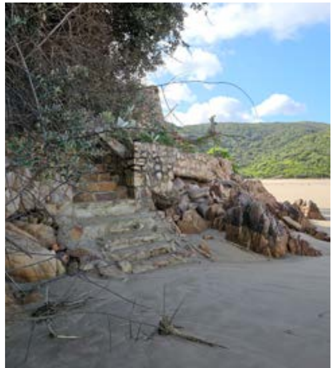
REPAIRED: Julie also employed a man to repair these steps, so that people could reach the beach, because the ramp from Wagon Road was washed away. The Steyns refunded Julie.
