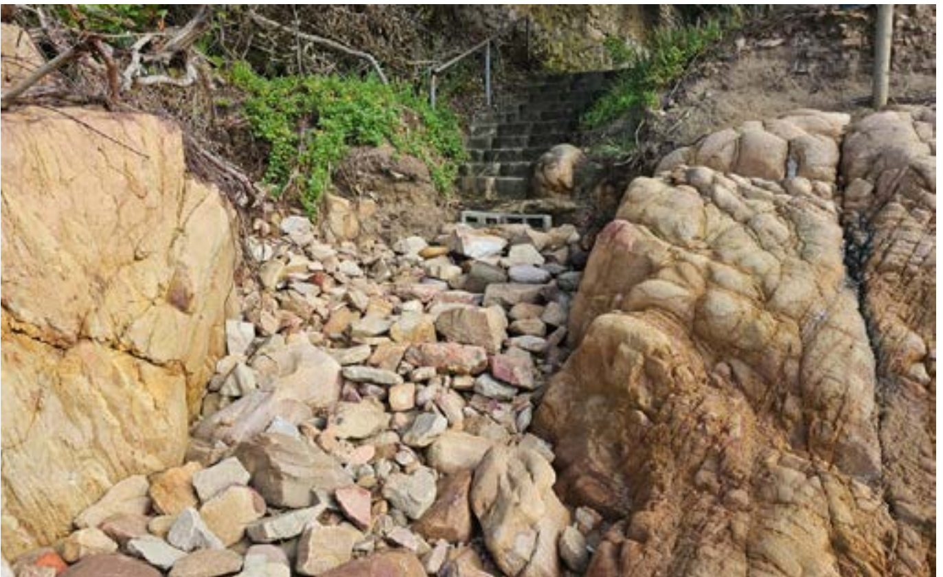
ROCKY: The 2024 storm surge scoured out the beach sand below the Municipal Steps, forcing visitors and residents to scramble over the rocks to get to the beach.
