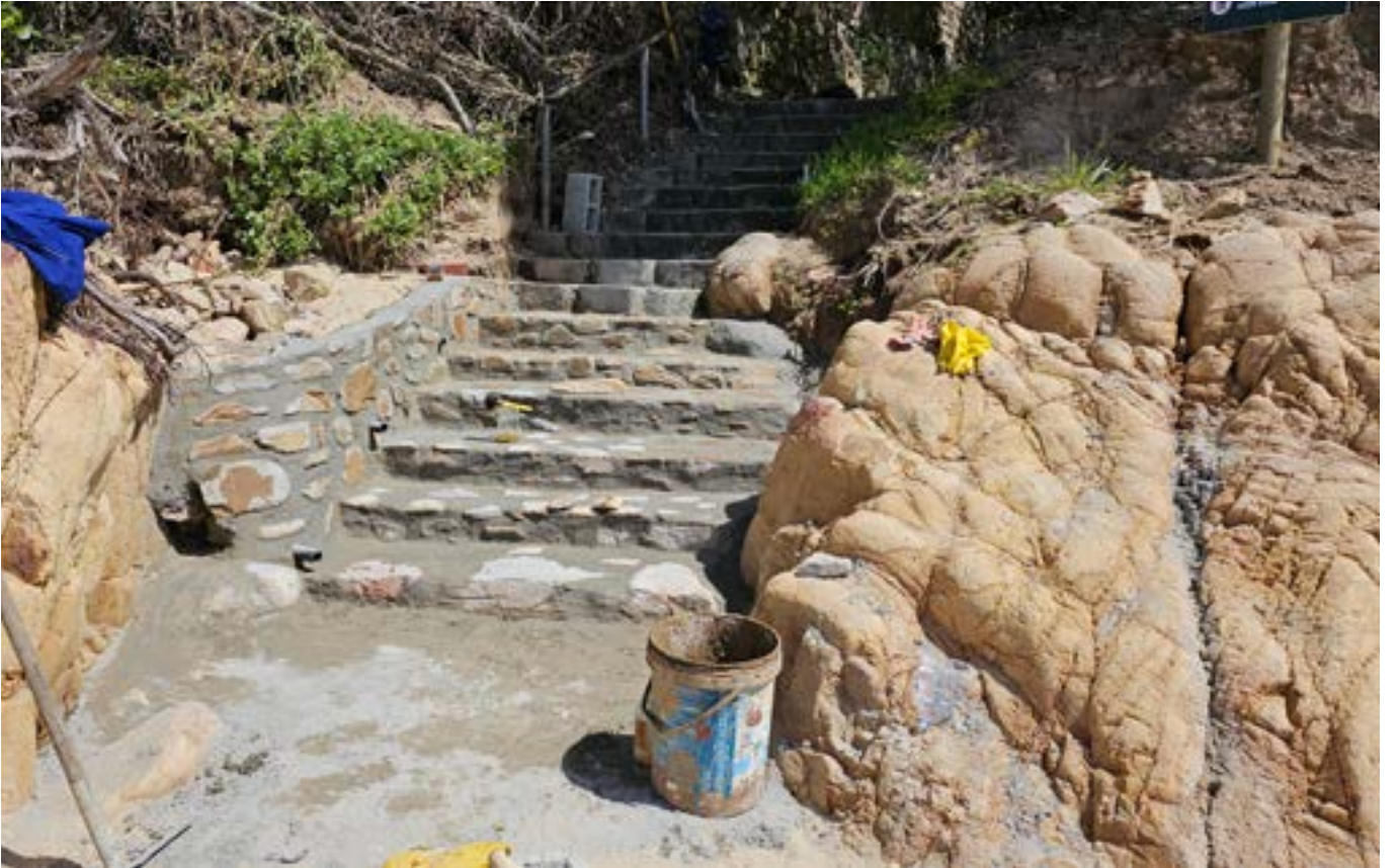
STEP EASY: The NCOA got permission from KM to repair the steps in terms of the MOA. The NCOA paid and Julie helped the builder to design them.
