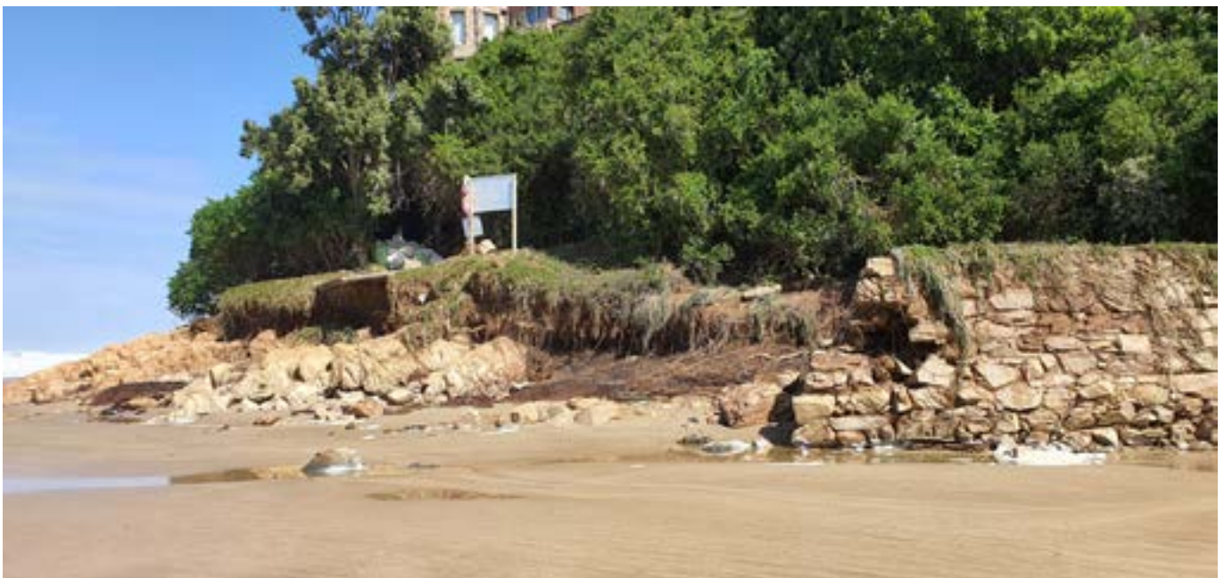
GOING, GOING...:The bank between the vehicle ramp and Wagon Road was badly eroded by both storm surges. Provincial engineers said further erosion could undercut the end of Wagon Road and prevent vehicles from reaching the beach.
