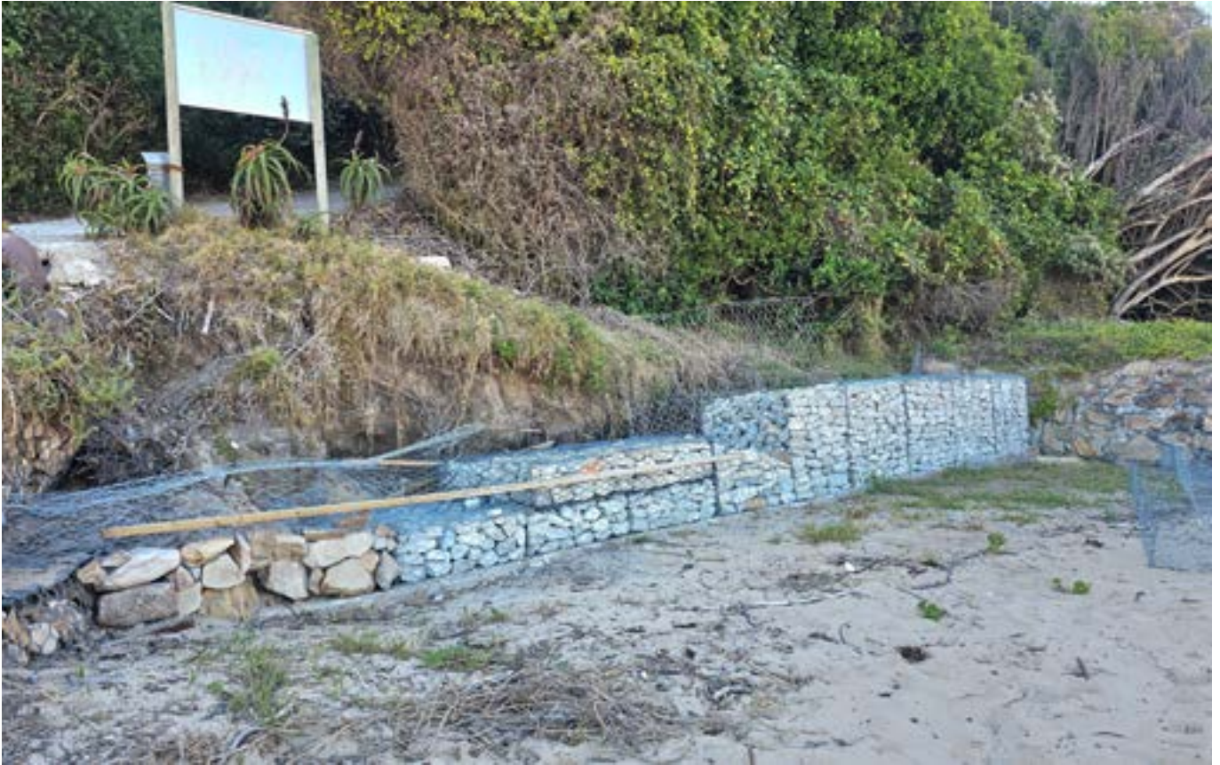
PROTECTION: A gabion wall, still under construction, will hopefully prevent further erosion of the bank adjacent to the old Wagon Road. This was paid for by national government disaster funding, topped up by Knysna Municipality.
