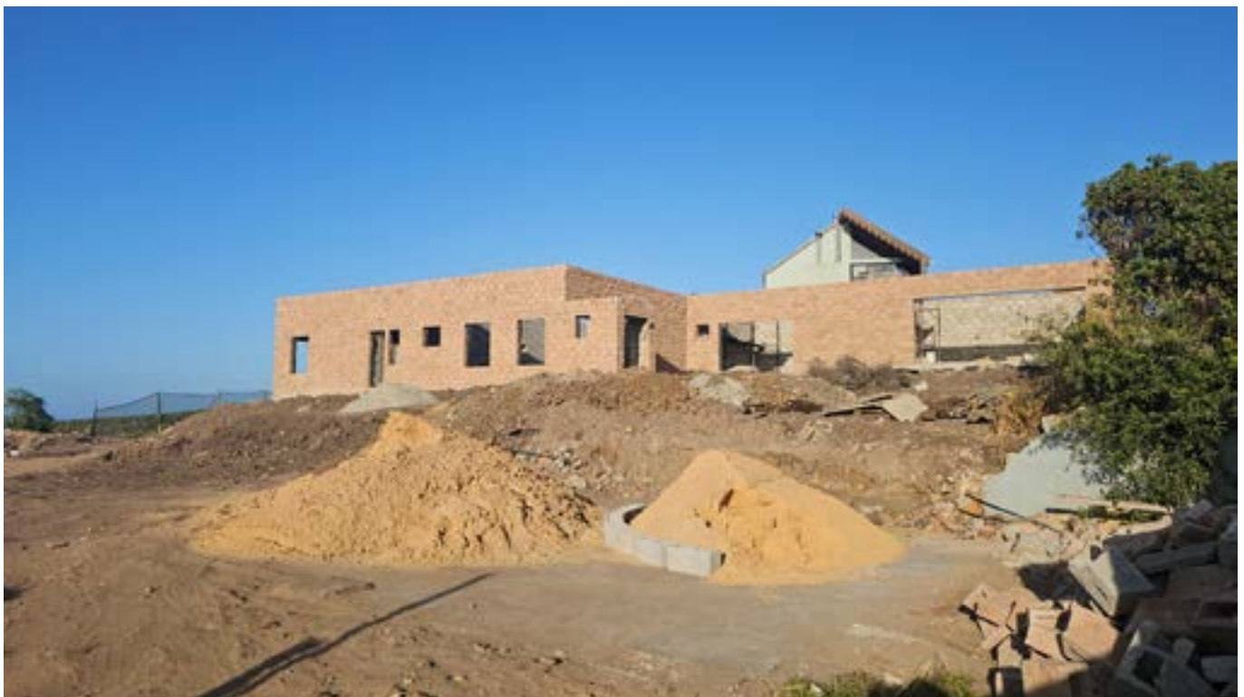
Bhyat house under construction on Noetzie headland.
